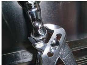
Fixing leaky taps, etc.
