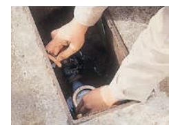
Replacing water meters.
