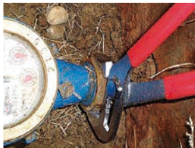
Plumbing & electrical work.
