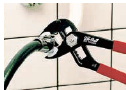
Fixing leaky taps, etc.
