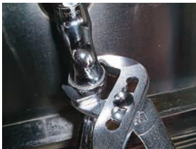
Fixing leaky taps, etc.
